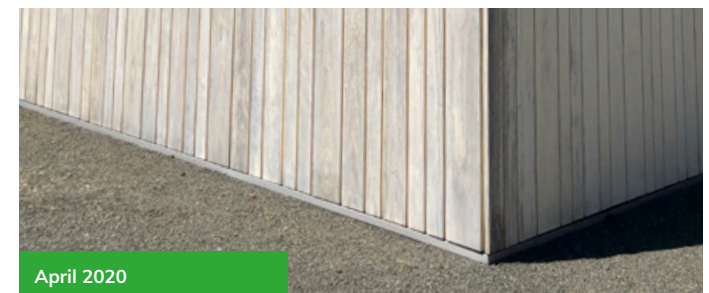
CLADDING PROJECT, NORTH AMERICA
